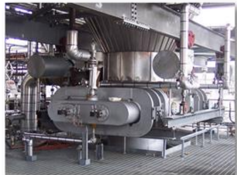
Completed Unheading Device Installation
